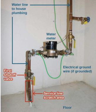
Identify a test area on the pipe between where the service line comes into the home (typically the floor) and the first shutoff valve. If the pipe is covered or wrapped, expose a small area of metal. Follow instructions in response to Question 2 to determine the pipe material.
